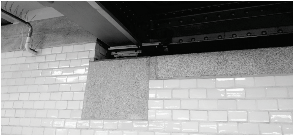
Fig. 7. Design assumptions and the final effect of lower bossages reconstruction.
