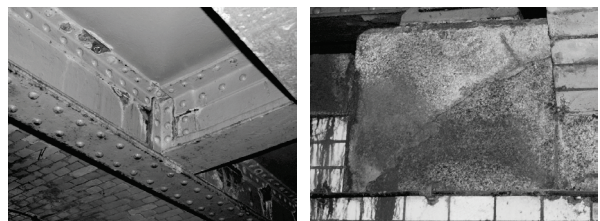
Fig. 4. Dyrekcyjna street passage: general view of the span, corrosion damage and cracking of the construction.
