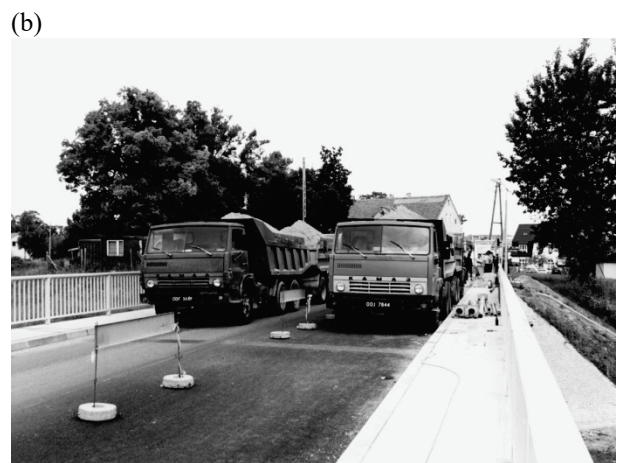
Fig. 4. Front view from Paczkow city centre on the span I loaded by: (a) two trucks (load scheme IN1) and (b) four trucks (load scheme IS) during field load tests.
