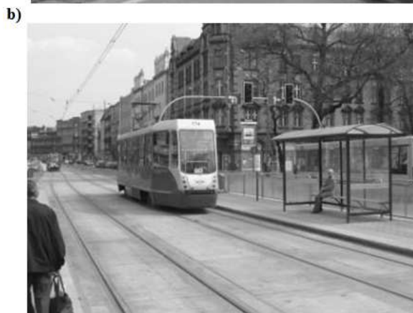
Fig. 11. Renovated tram platform with traffic lights at 3-go Maja street in Katowice.
