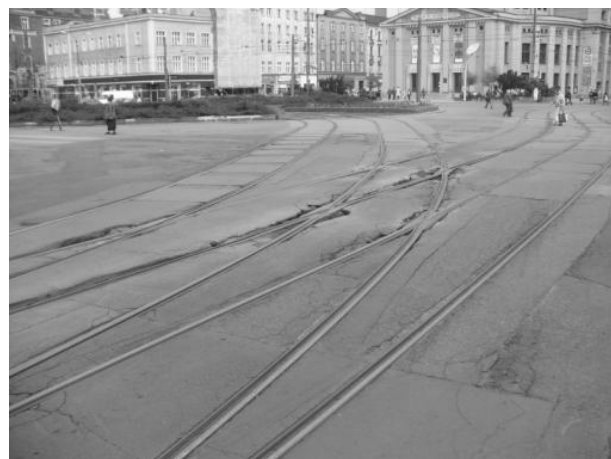
Fig. 10. Tram trackway at Katowice market place.
