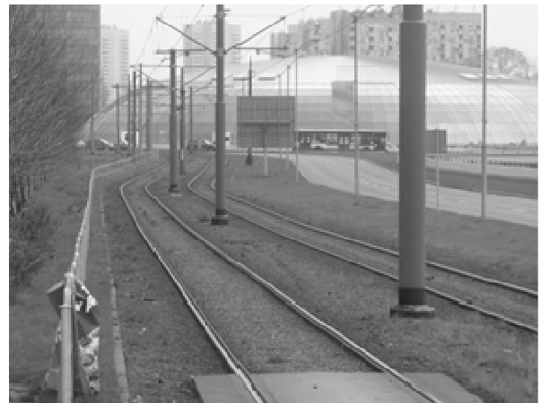
Fig. 5. Separated tram trackway. Chorzowska Street in Katowice Source: own elaboration
