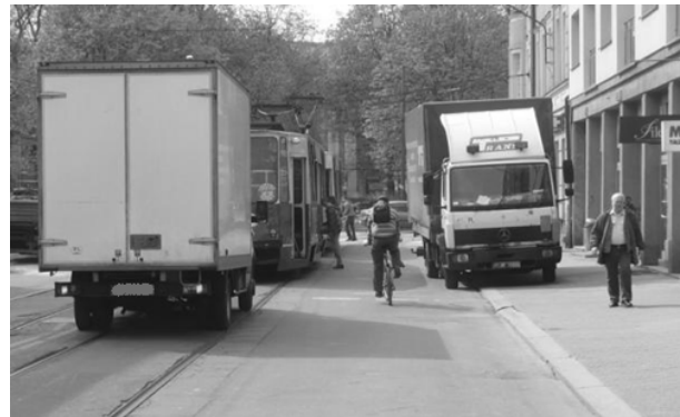
Fig. 9. Tram stop without safety island at 3-go Maja street in Katowice.
